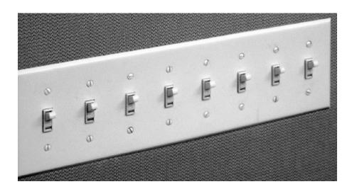
**FIGURE 4.4. Incomprehensible Light Switches.** Banks of switches like this are not uncommon in homes. There is no obvious mapping between the switches and the lights being controlled. I once had a similar panel in my home, although with only six switches. Even after years of living in the house, I could never remember which to use, so I simply put all the switches either up (on) or down (off). How did I solve the problem? See Figure 4.5.
